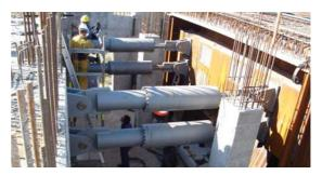
Fig. 31: Dampers (MHD) installed in a brdige
